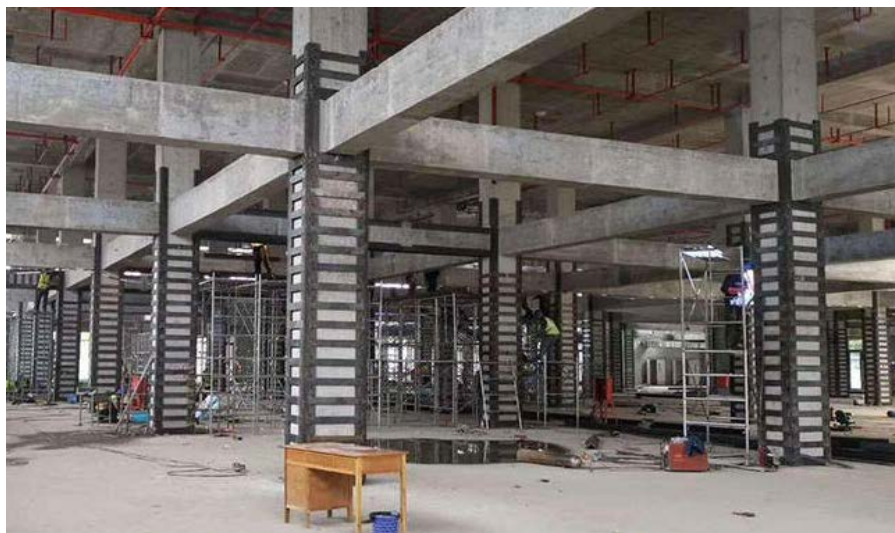
Figure 2. Steel jacketing of column
